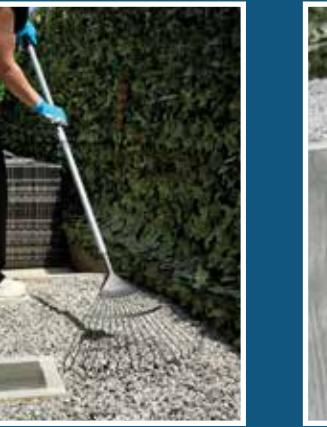
After applying the first coat, rake or move the rocks to expose the uncoated material. This ensures that the surface is sufficiently covered with EASIHOLD.
