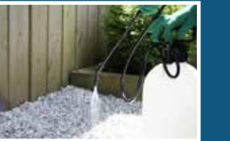
Apply the first coat to the clean dry surface, spraying slowly and in a controlled manner, ensuring even coverage.
