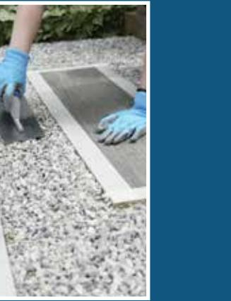
For the second coat, follow the same method as in phase 2. Once uniform coverage is achieved, compact the surface to obtain the best adhesion result.
